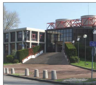
The IN2P3 Computing Centre operates a Tier-1 site for the LCG.
